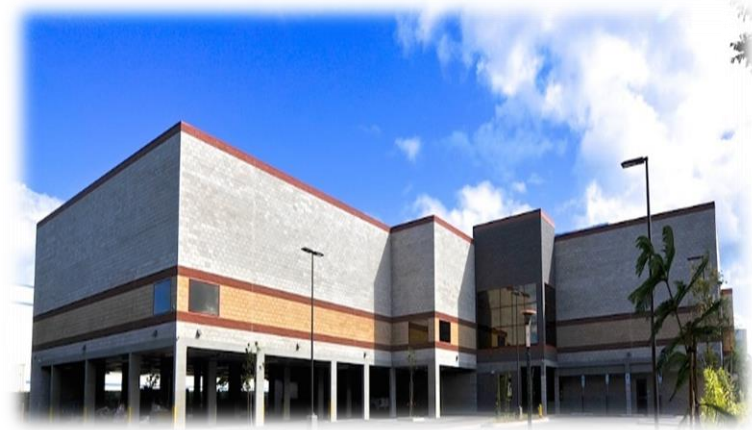
8-inch masonry walls range from 30-40 feet in height
