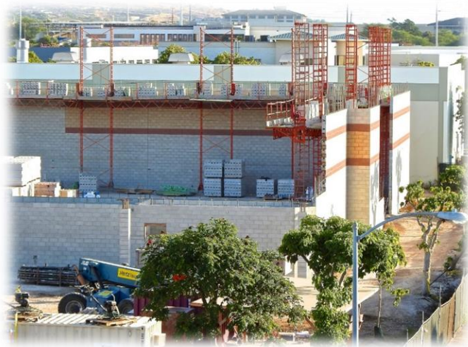
808 FUTSAL built in 24 months using 8" CMU
