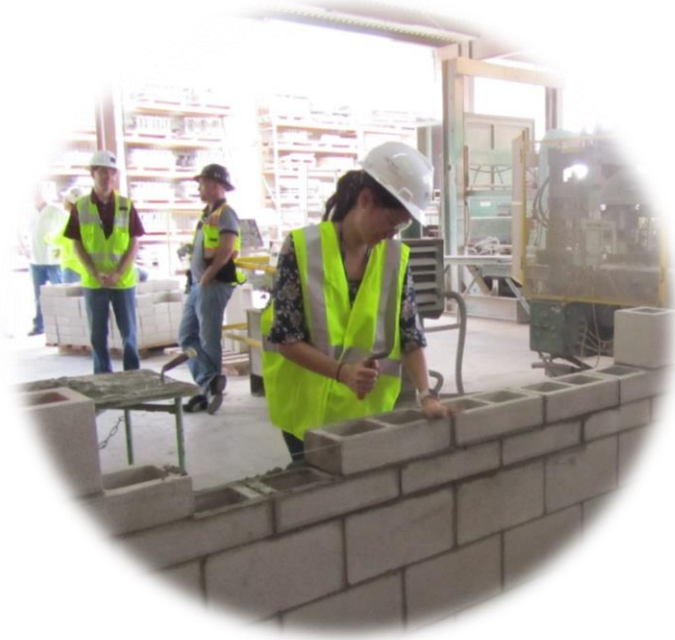
Hands-on setting CMU blocks
