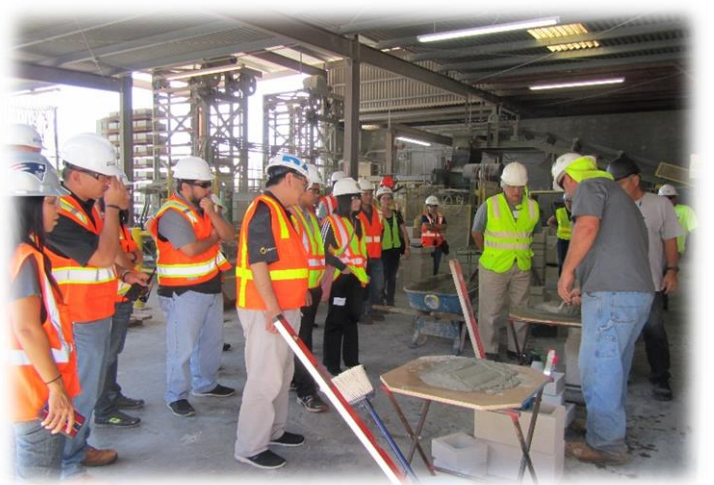
Quality General's masons provides demonstration on mortar
