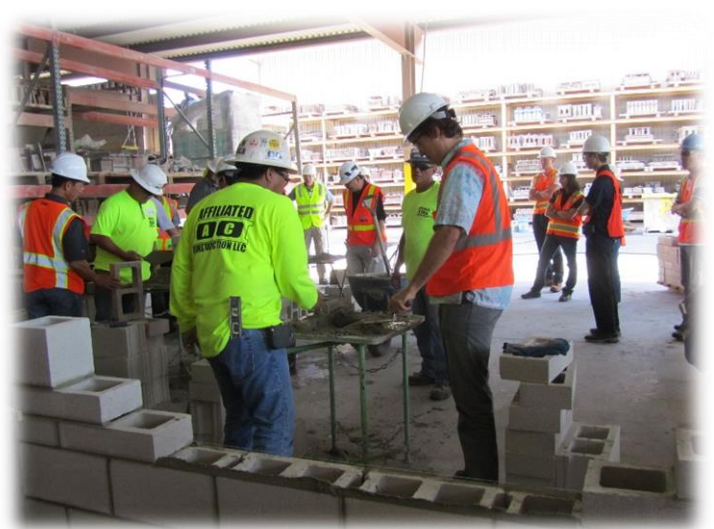
Affiliated Construction's masons mixes cement mortar
