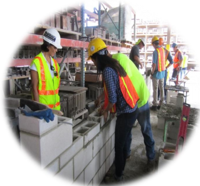
Women at work setting CMU Blocks
